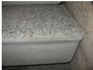
Exposed Aggregate Finish
